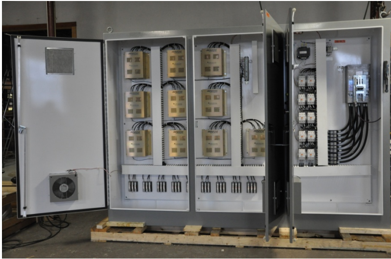
Left and below left: 10 Zone 800 Amp System for PECO experimental wind turbine power station.
