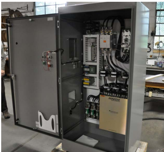
Below: 480V 350A 3 Phase transformer primary driver. System has remote power monitoring transducers, as well remote command and control signals to and from a PLC. System used outdoors, NEMA 4 w/ Air Conditioning unit. Petrochemical application.
